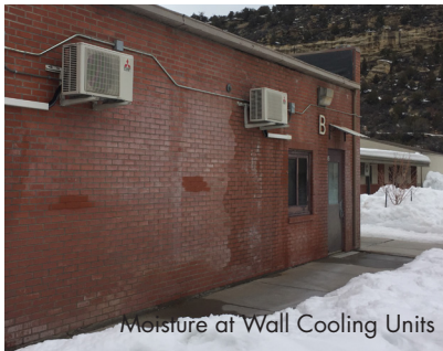
Rotting Brick at MS
